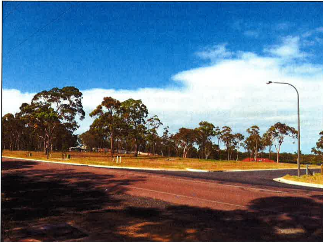
Figure 2 Subdivision Works (former Lot 1 DP 555602)
